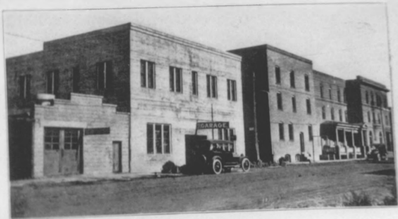
The Olive Garage and Repair Shops.
